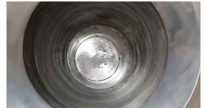
Photo of cladding inside the body of the 20inch-2500# GATE VALVE
