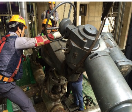
The VALVE MEDIC TEAM (valve maintenance organization) is repairing the MOTER OPERATED VALVE.
